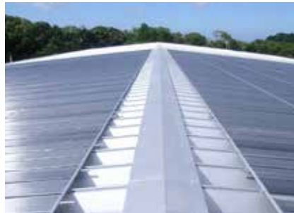
Roof shades(Kikugawa South Factory)
