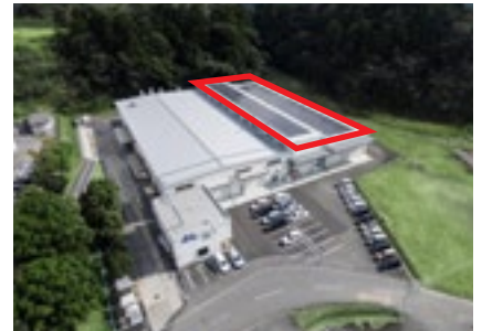
Solar Power Facility of Star Metal Company (Red flame)
