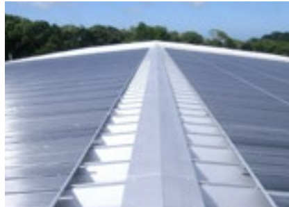
Roof shades(Kikugawa South Factory)
