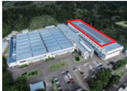
Solar Power Facility of Kikugawa Factory (Red flame)
